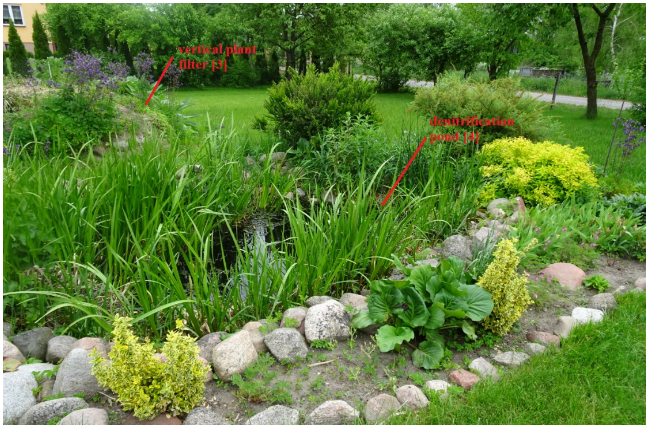
Figure 4. The elements of domestic wastewater treatment plant in Idzki-Wykno village [own photo, 06.2017]
