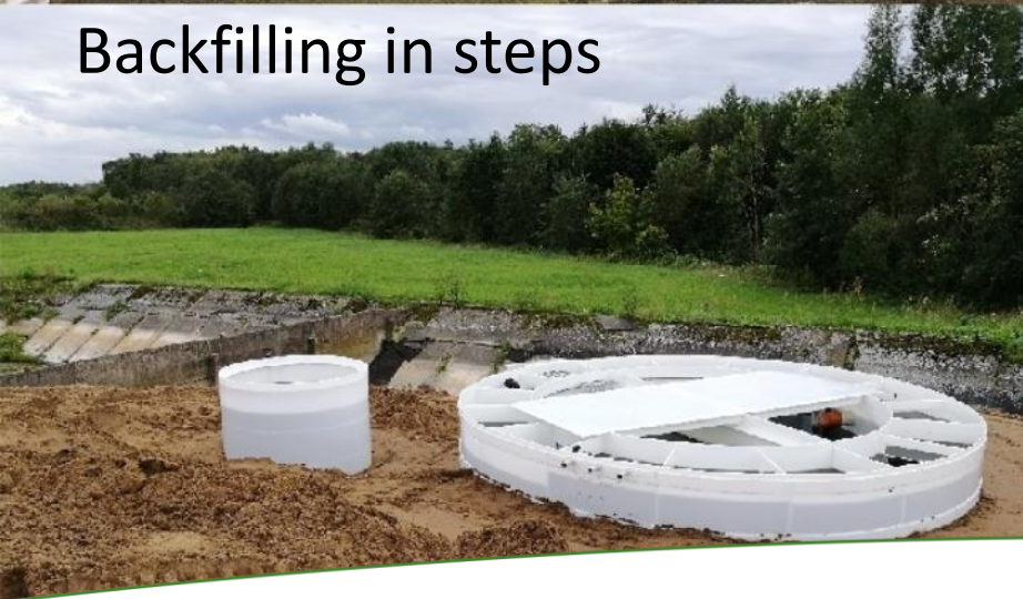
Last step, after connecting the piping
