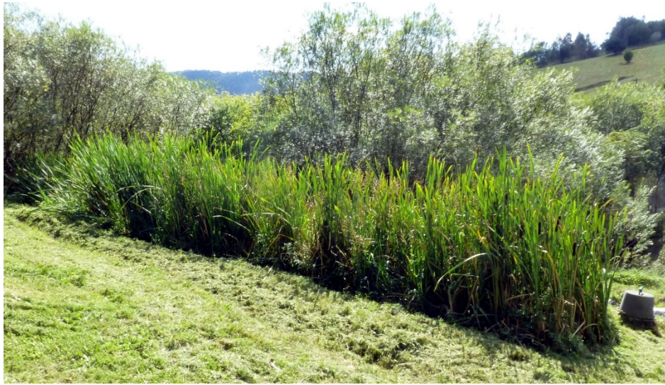
Shallow ditch planted with Typha latifolia for final wastewater treatment
