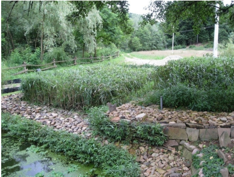
An example of household wastewater treatment plant in the form of a cascade of filtration beds filled with gravel, sand, soil and hydrophilic plants, according to ITP ZSIT GCB Tylicz project.
