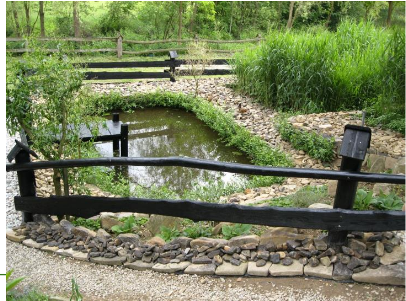
Another example of garden pond (micro-retention of treated effluents)
