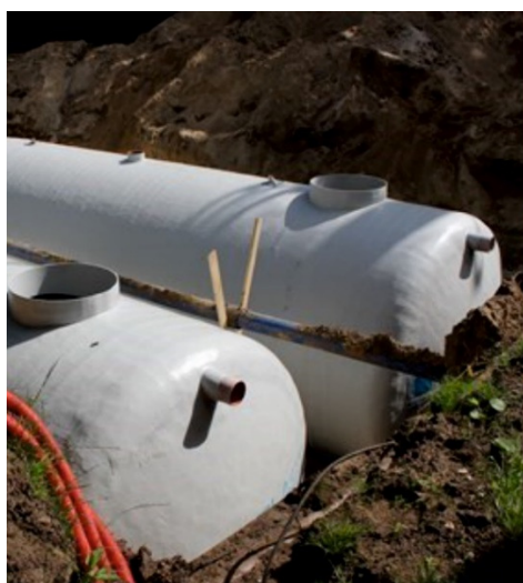
Figure 6. Wastewater holding tank with filling alarm. Photo: Scan-Plast Latvia LSEZ SIA
