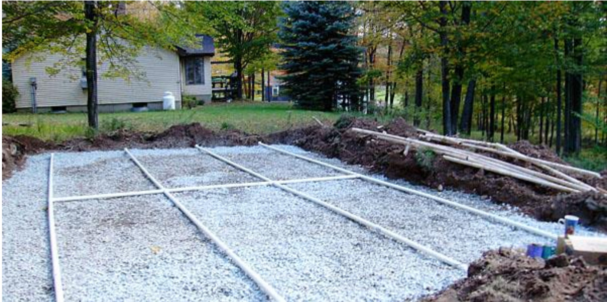
Figure 18. Traditional infiltration field under construction. (Source: www.koberlein.com )
